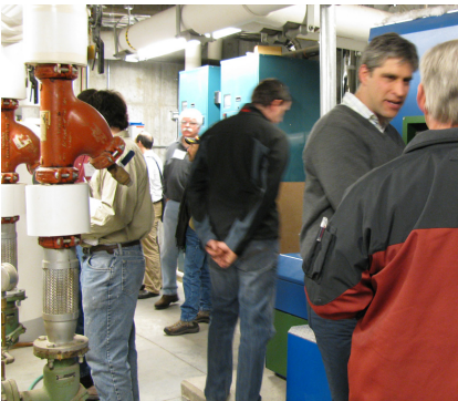
David Dungate of ACT Bioenergy (right, facing camera), gave a tour of The Wild Center's system, the first commercial scale pellet boiler in New York State, during the April 19 Biomass Basics workshop. Dungate designed the boiler, which saved $31,652 in its first year.
